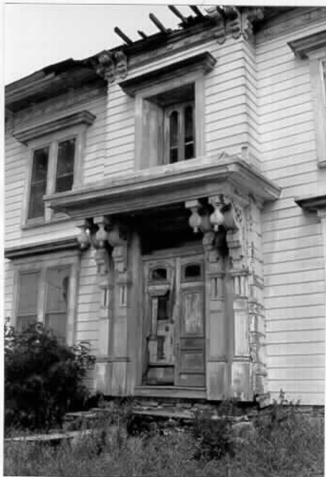
5. Salvaged interior woodwork
