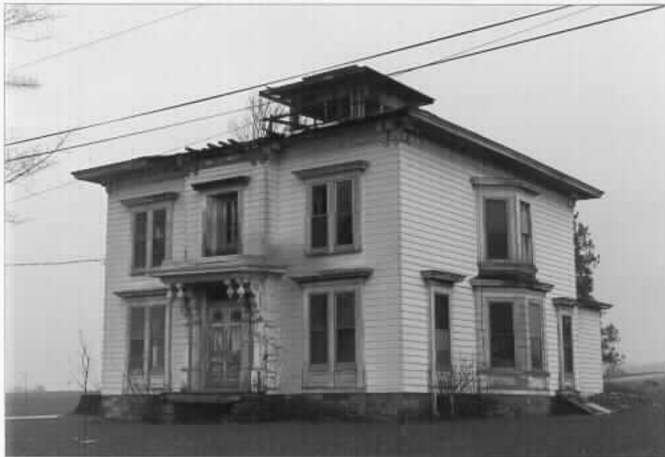
2. Farmhouse, viewed from southeast
