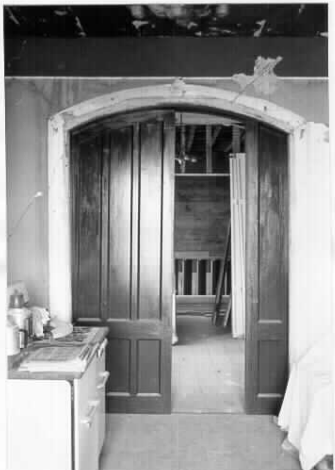
9. Pocket doors between southwest and north- west parlors
