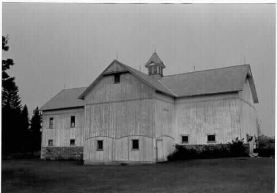
11. Barn, viewed from southeast
