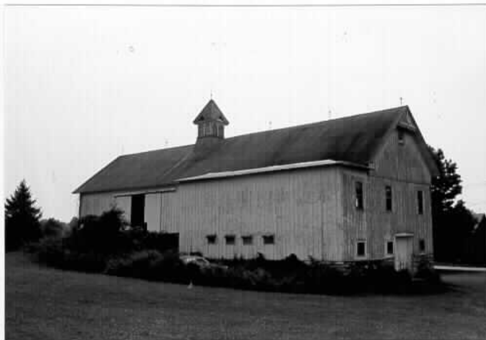
13. Rear elevation, viewed from northwest
