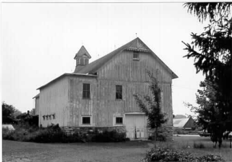
12. Barn, viewed from west
