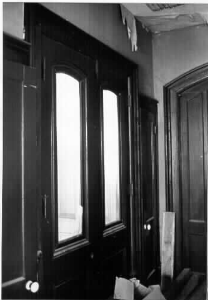
8. Door detail, entrance parlor
